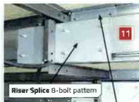
Nosebeam Splice 4-bolt pattern
